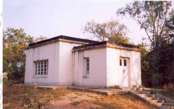
Fig. 2.1.3: Secondary variometer building (GEOMAG-02M+GSM19)
