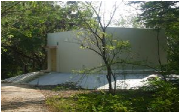
Fig. 2.1.2: Primary variometer building (DFM system)
