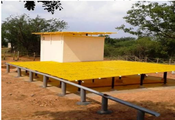
Fig. 2.2.1: Primary variometer building (DFM)
